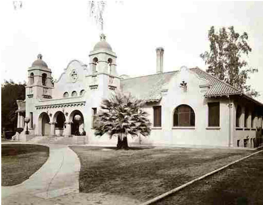
Figure 9. Riverside’s Carnegie Library (1903-1964), designed by Arthur Benton, exemplified the architectural motifs characteristic of the Mission Revival style. The design is fundamentally ecclesiastical, presumably to suggest that the library was a temple of learning. This metaphor was one that Andrew Carnegie specifically encouraged in libraries he funded. The steps leading to the entrance (visible on the left) symbolized personal elevation, and the lamps alongside the steps represented enlightenment. (Riverside Public Library, Photo LIB RIV CEN CAR V 22 CLD2-98)
